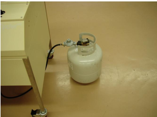
Figure 2.2: 20 lb. Propane Cylinder with Regulator
